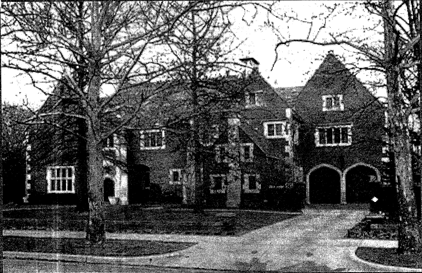
$170 K College Hill - major slate roof repair and HVAC system
