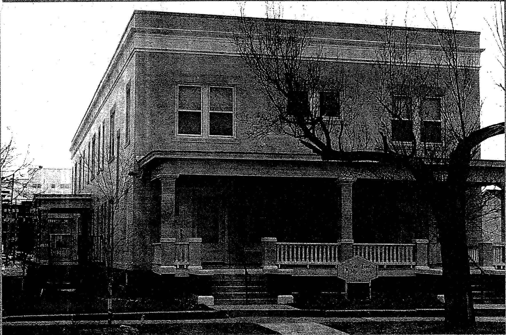
$900 K rehabilitation for affordable housing units
