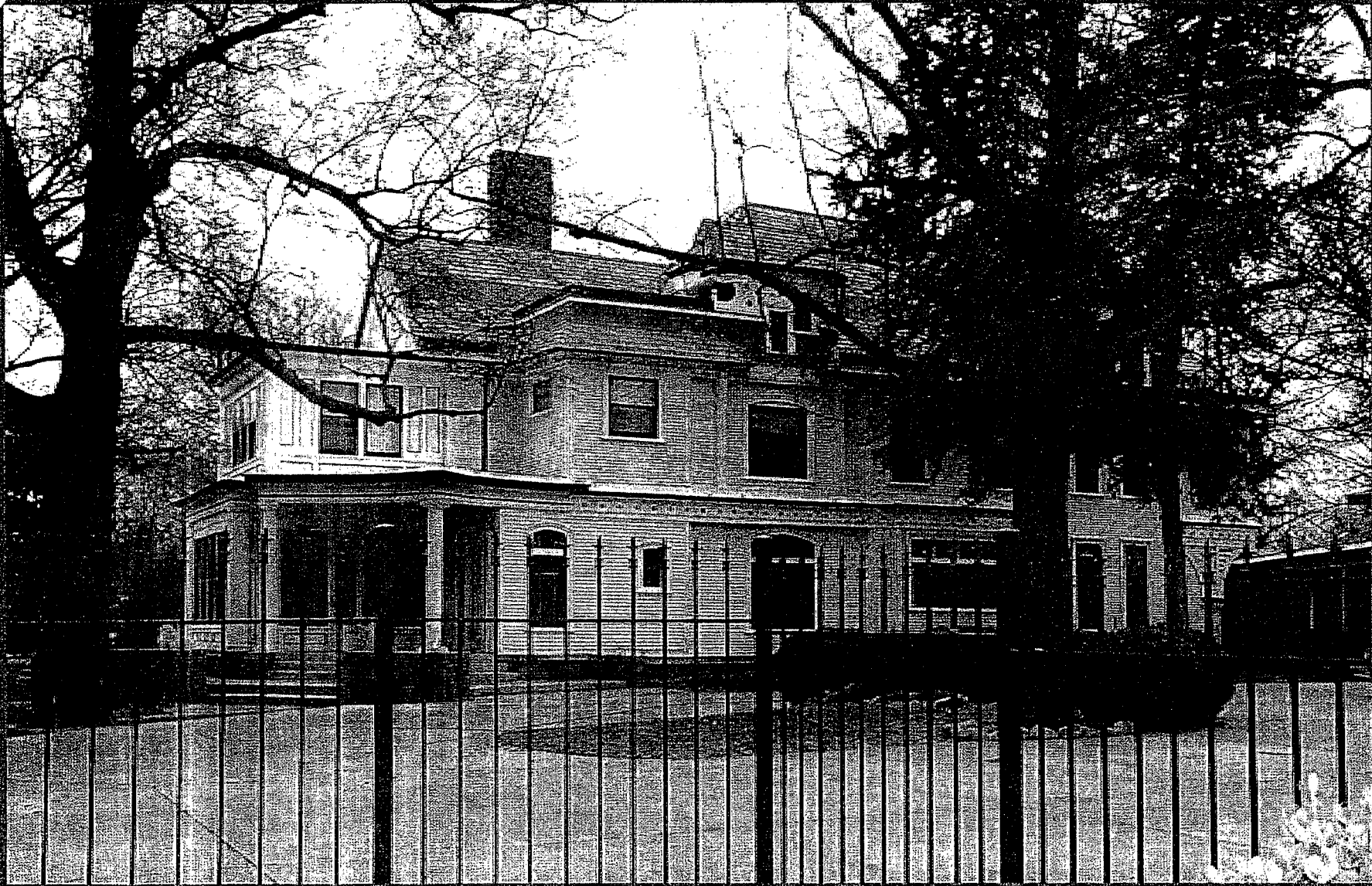
$460 K rehabilitation - LW Clapp House
