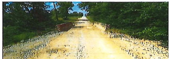
Lookout Road South of 287th, Bridge I-14.1
