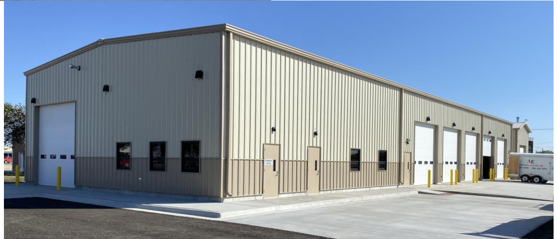
Clay Center After
