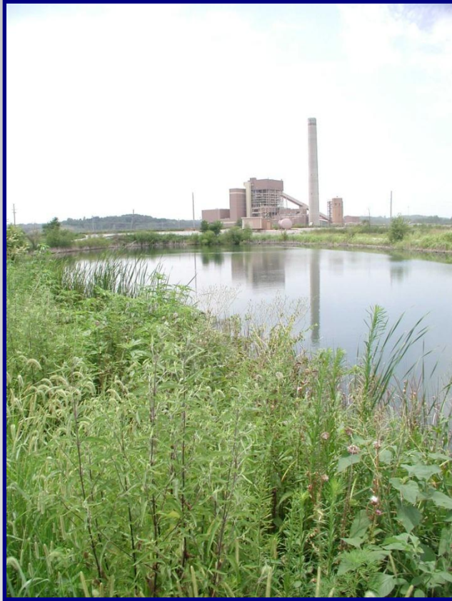
Nearman Creek Power Station
